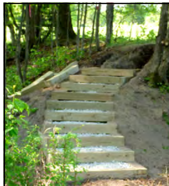
Steps under construction
